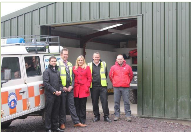
Aberglaslyn Mountain Rescue Base was refurbished thanks to CCG contractors GM Jones, Falconer Electricals and suppliers, Travis Perkins.
