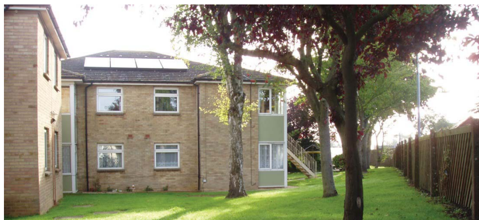
Sustainability issues, photovoltaic cells installed by one of CYNTRA's contractors
