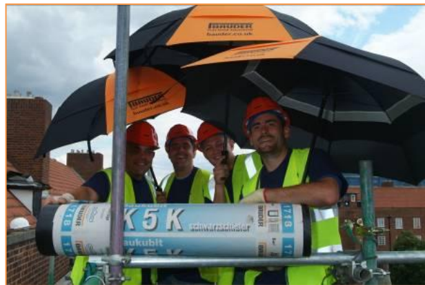
Continuity of work meant continuity of labour on site resulting in consistently high quality workmanship
