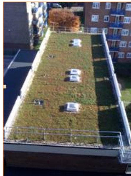
Green roof material donations for trial projects such as Tradescant House on the Frampton Park Estate, Hackney. This allowed Hackney Homes to help residents understand the aesthetic, environmental and economic benefits of installing green roofs
