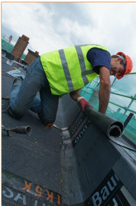
Roof installation at Hackney
